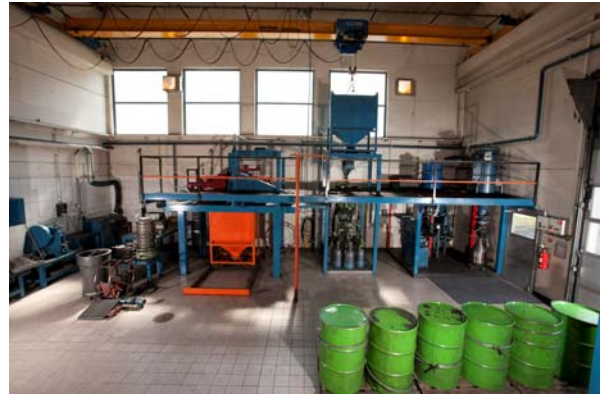
Figure 3: Pilot plant to prepare dry aggregate
