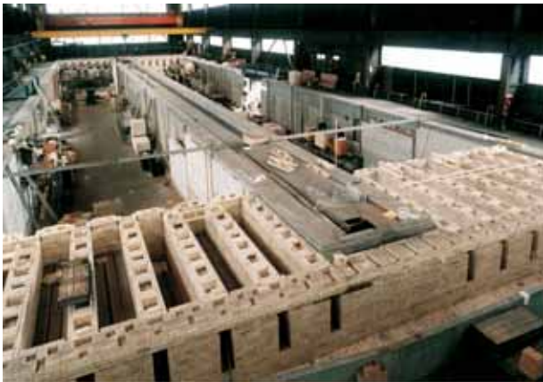
Figure 1: Open top ring type furnace under construction
