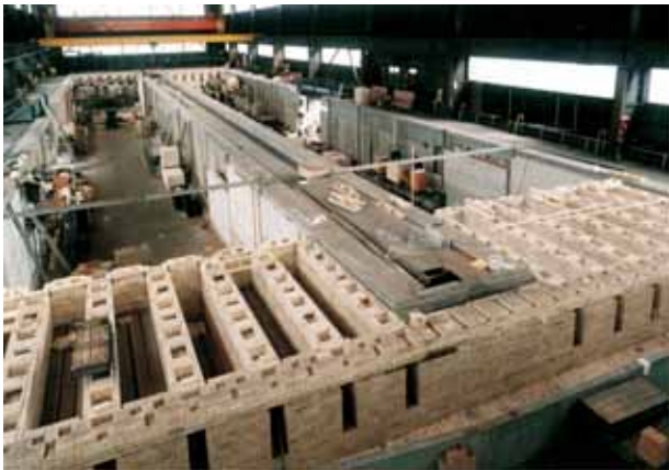
Figure 1: Open top ring type furnace under construction
